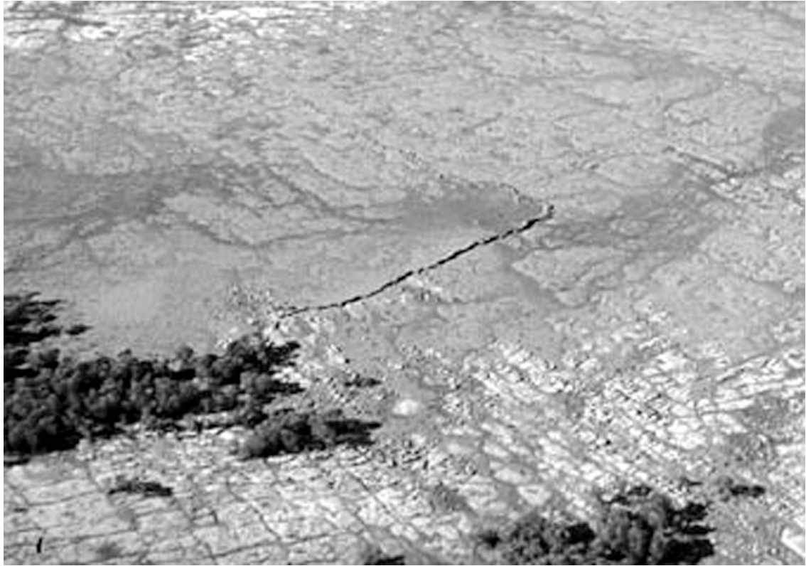
Figure 5.8: Trap wall designed to take advantage of a rocky substrate and a drainage channel system. (Photo by Errol Stock, July 2004.)
