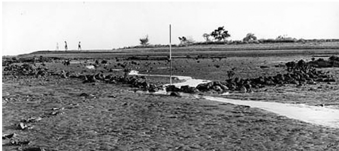
Figure 5.7: Trap wall at low tide, showing a drainage channel and indicating a likely point to design in a gate. (Ref. RB 5668/7, AERC L8/2-158).
